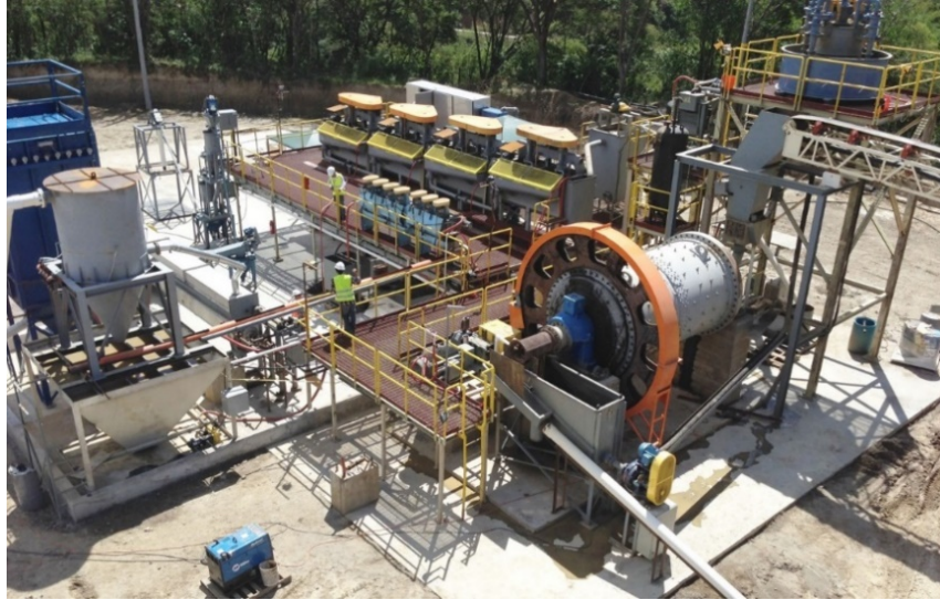
Figure 5 Tambor flotation plant 119
