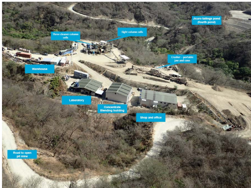
Figure 6 Tambor plant area 120
