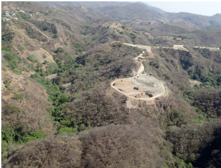
Figure 10 Poza del Coyote pit 137
